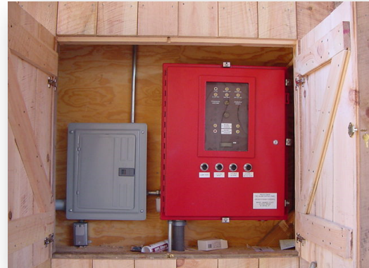
Protectowire Cabinet (Slate Covered Bridge)
