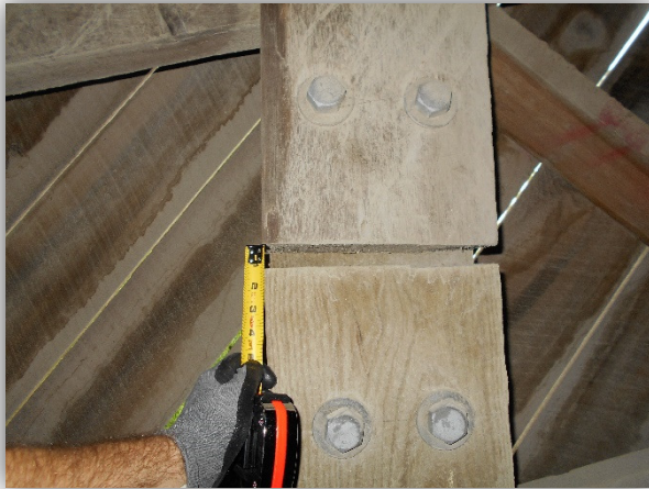
Typical Gap at Spliced Lattice Members
