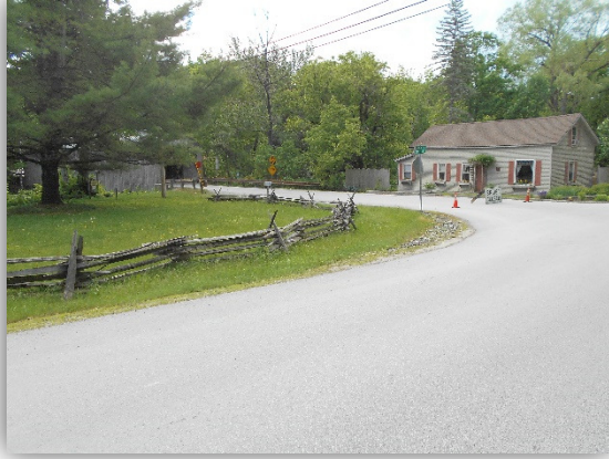
Stone-Lined Drainage Swale at Intersection
