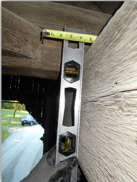
Out of Plumb Chord 1 South End of West Truss
