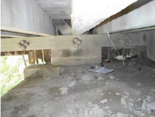
Existing Bearing Blocks
