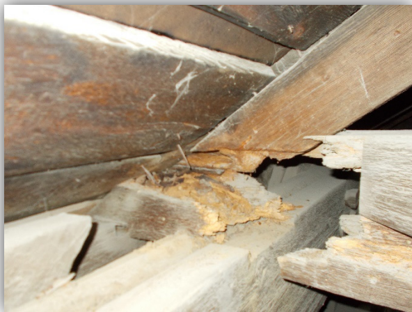
Heavy Rot at Cross Beam Node 10/11 West End
