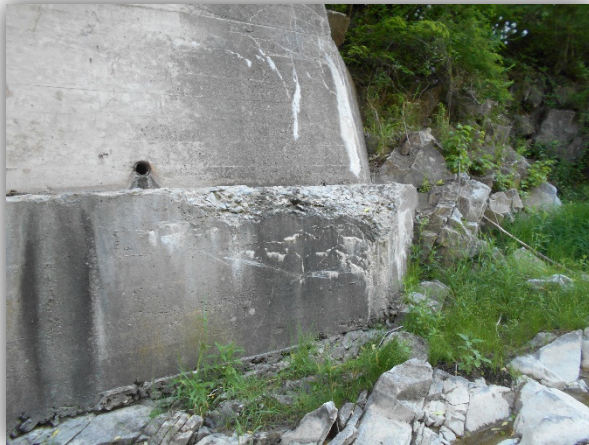
Abutment No.2 (North) Footing Spalling and Efflorescence Staining
