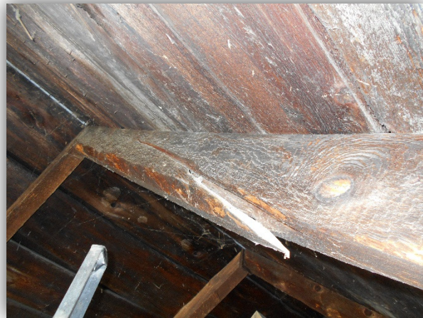
Typical Broken Roof Rafter
