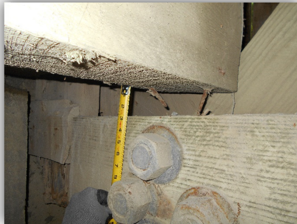
Floor Beam to Chord 4 ½" Gap Due to Bearing Block Extensive Rot – South End West Truss
