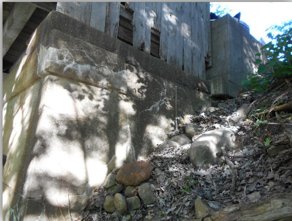
Wingwall No.1 (Southwest) Undermining
