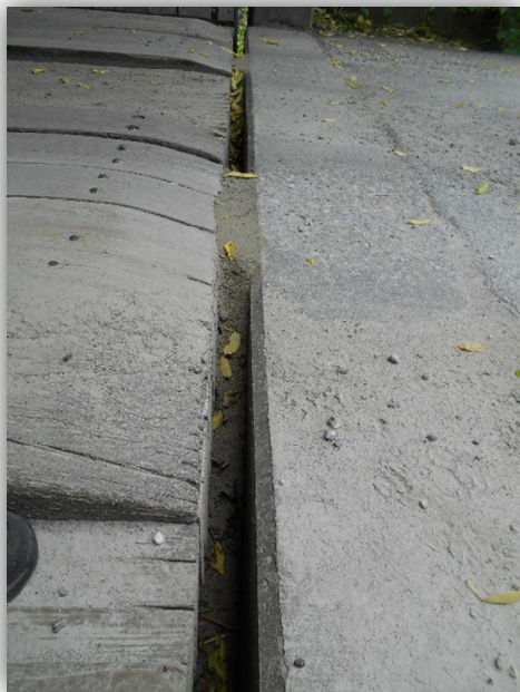
Tapper Runner Boards at Abutments
