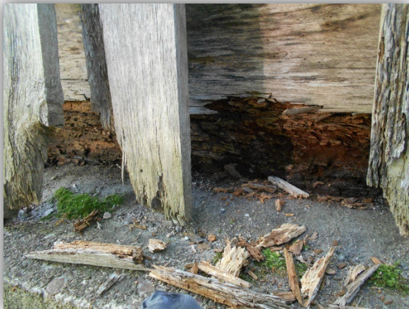
Bearing Block Rot South End West Truss
