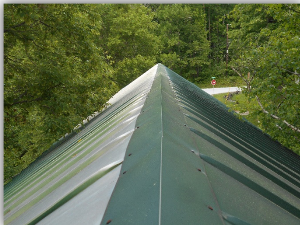
Nailed Ridge Cap Metal Roof Paint Failure – Left Side
