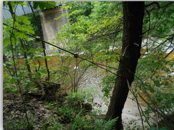
Typical Guy Rod Tied to a Tree
