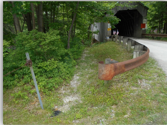
Existing W-Beam Guardrail and Drain Pipe
