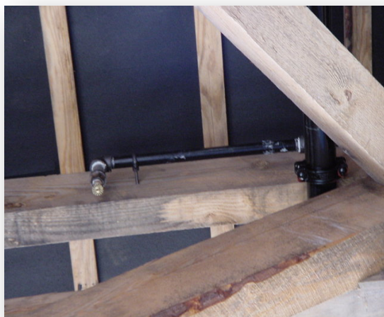
Typical Sprinkler Head (Slate Covered Bridge)
