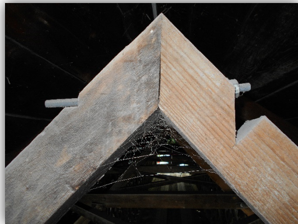
Typical Broken Roof Rafter
